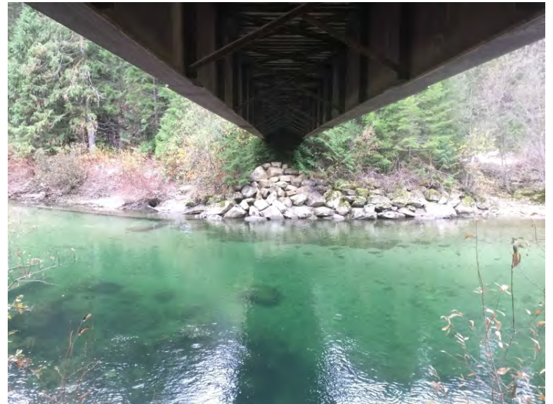
Right Bank Abutment when facing downstream
