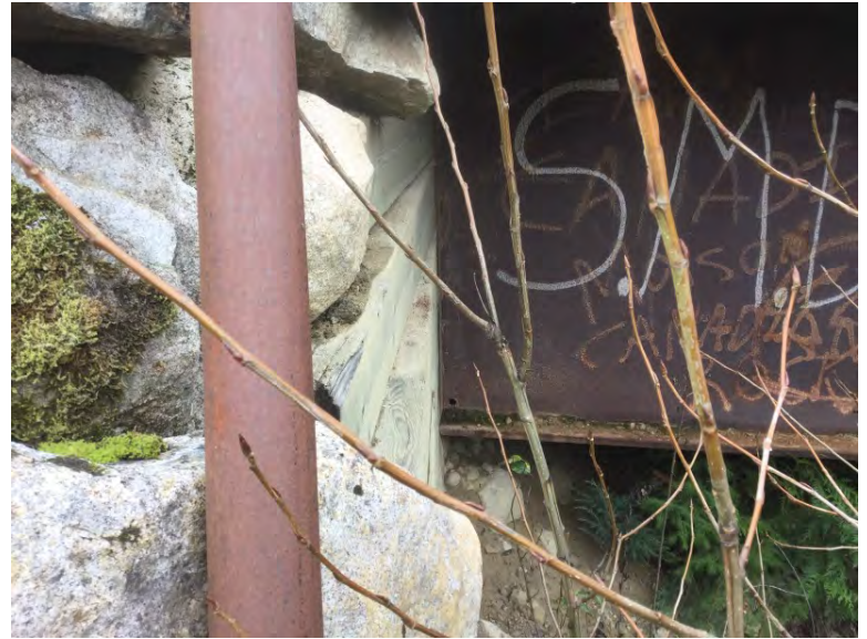
Left bank ballast wall
