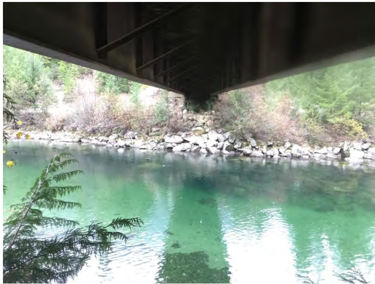
Left Bank Abutment when facing downstream
