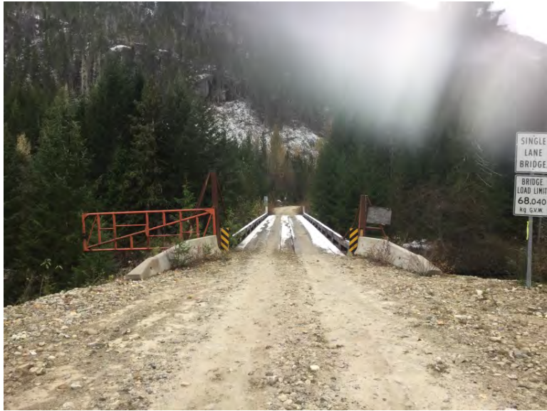
Approach from Left Bank when facing downstream
